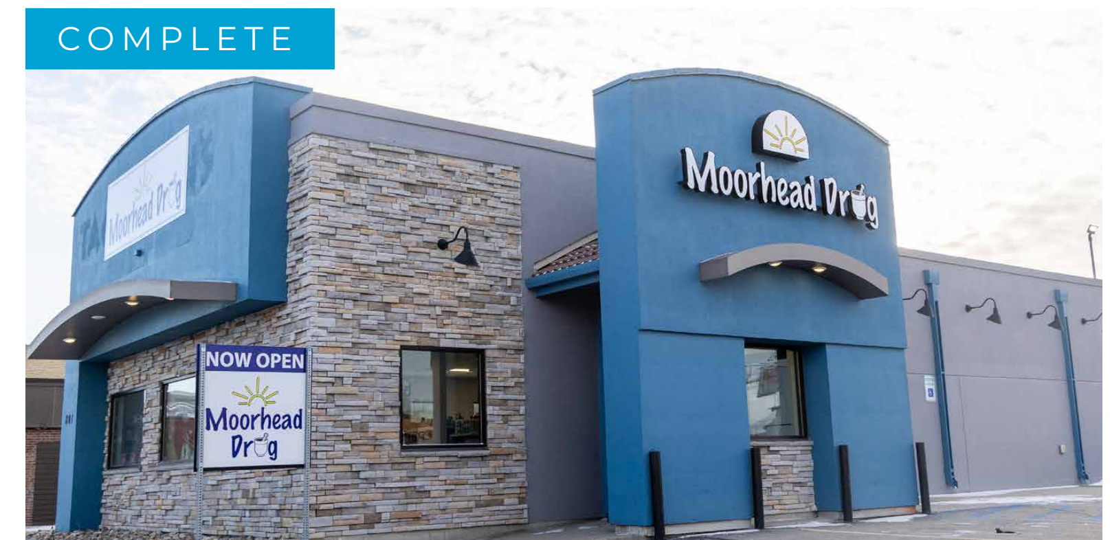
COMPLETE Moorhead Drug » 801 Center Ave Pharmacy relocation and renovation
