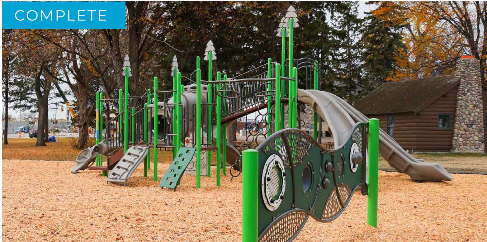
W.H. Davy-Memorial Park » 111 8 St N New park facilities installed
